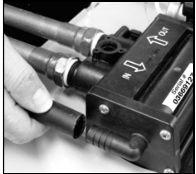
Figure 3 CONNECTING DRAIN LINE
