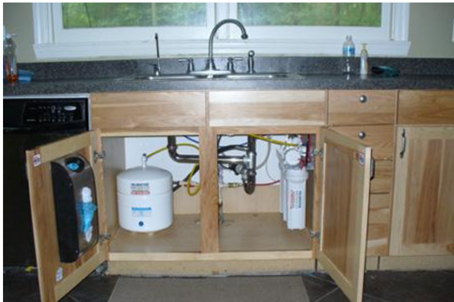
Standard 5 Stage Reverse Osmosis System - home under sink
