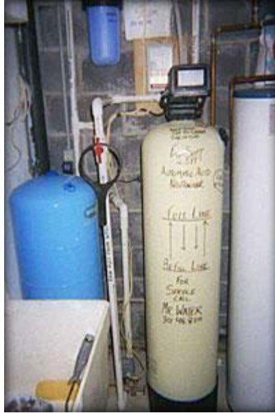
Acid Neutralizer to prevent green staining of fixtures and corrosion of copper piping. This system has a post filter for taste and odor. Installed in Ijamsville, MD 21754.
